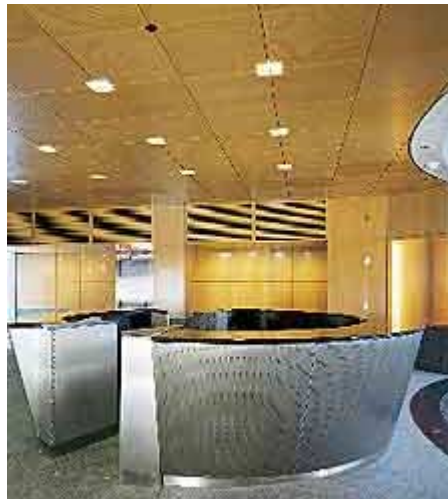
A custom beech perforated-wood ceiling was used in conjunction with non-woven acoustical fabric for this office space in Los Angeles.
